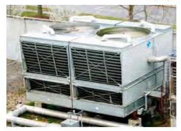
Min. 5 cycles of concentration when potable water is used
